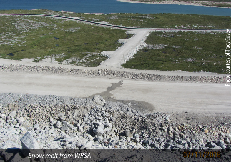
Type 1 rock that will be used as to cover the WRSA
