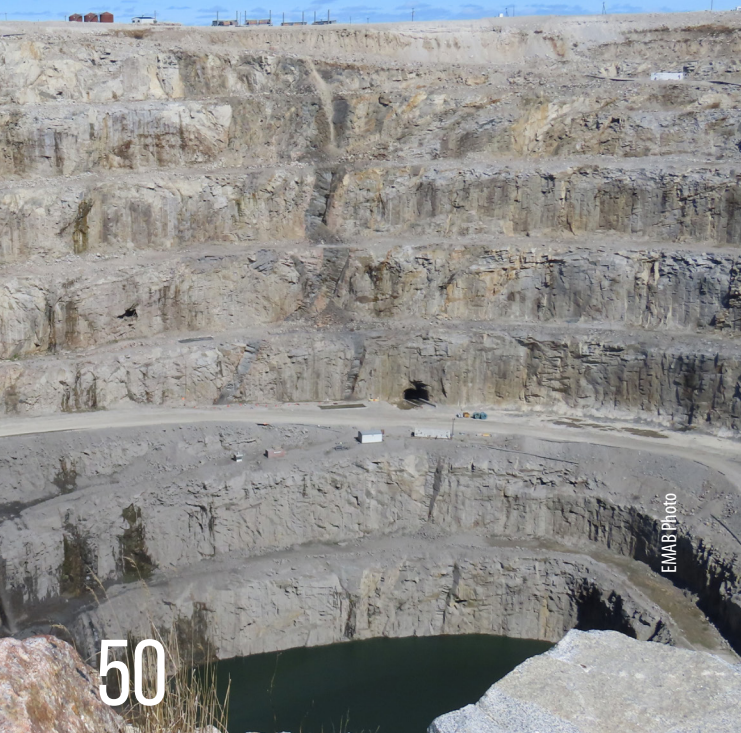
A418 pit being filled with processed kimberlite slurry
