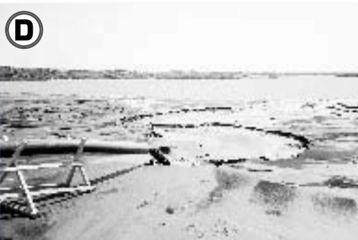
Outflow from process plant to processed kimberlite containment facility.
