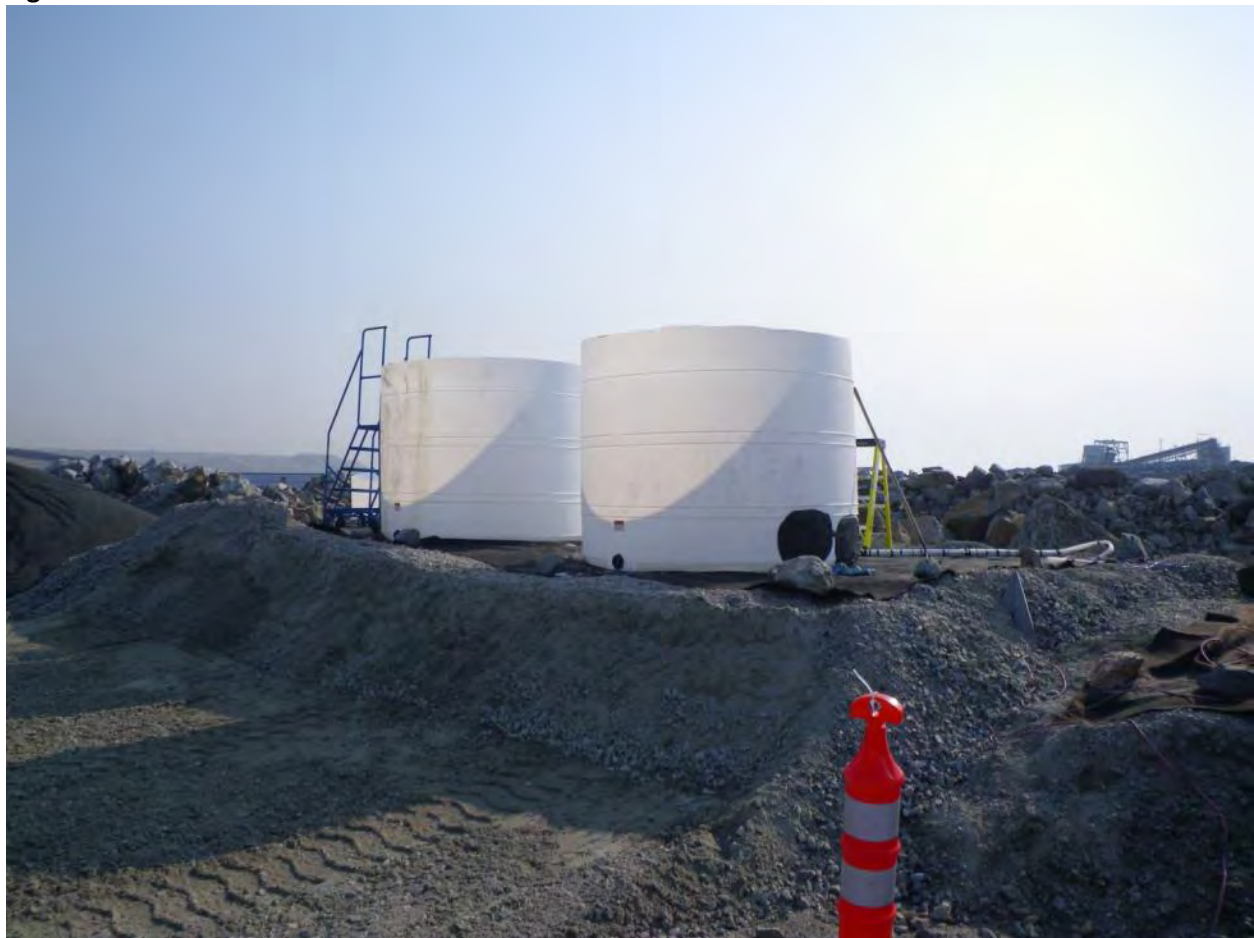
Fig. 2. CPK tanks before CPK and instrument installation
