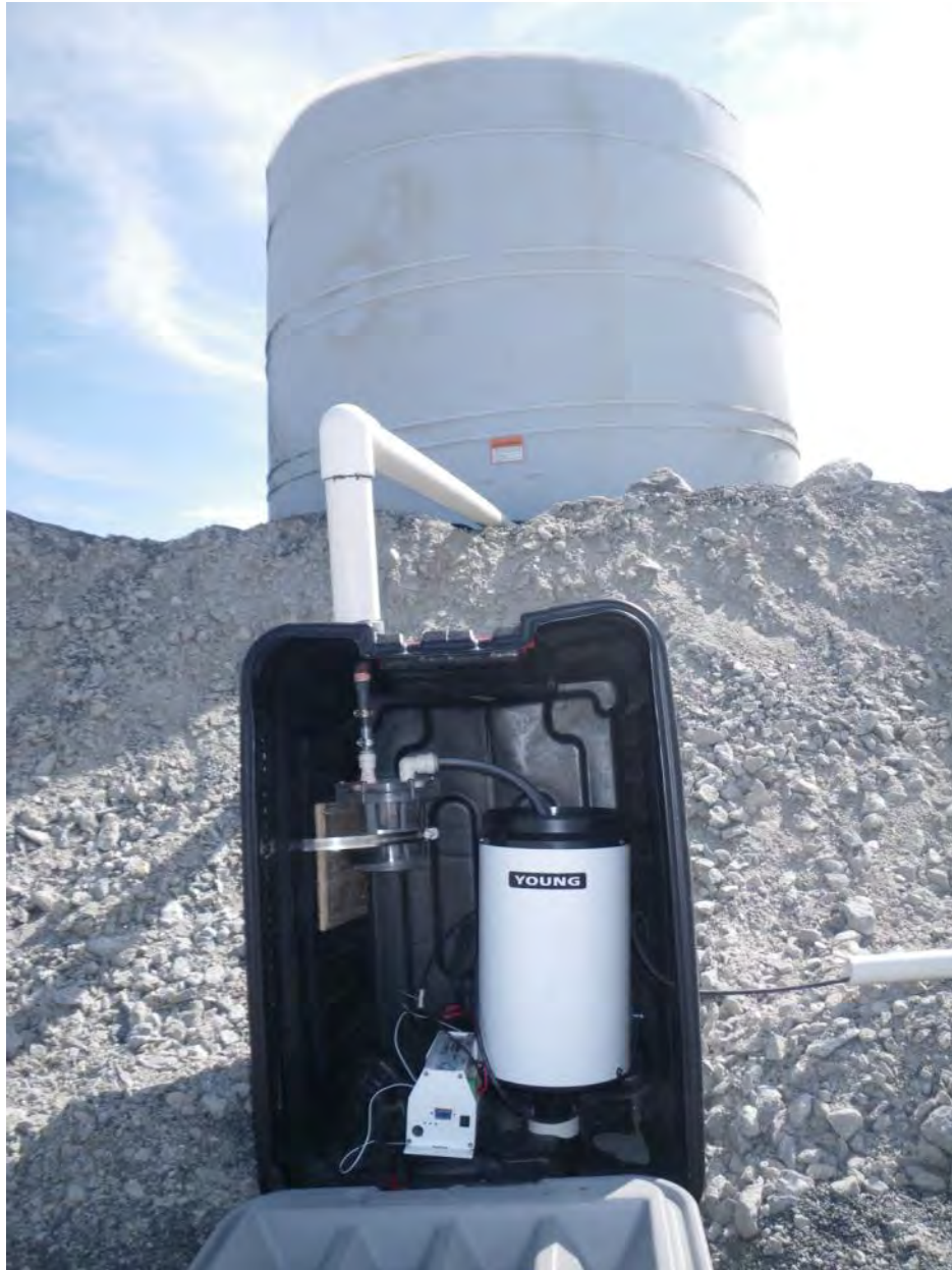
Fig. 6. Completed drain line from tank directing flow to sample cell and tipping bucket flow gauge. Tipping buckets from both CPK tanks are wired to one Data Dolphin datalogger.
