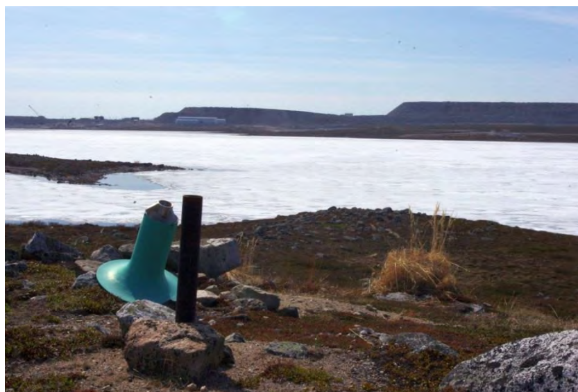
Photo 2: Fiberglass Shield Removed
