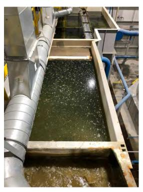
The water treatment plant is equipped to treat 90,000 m³ of water per day, some of which is pictured in settling ponds.
