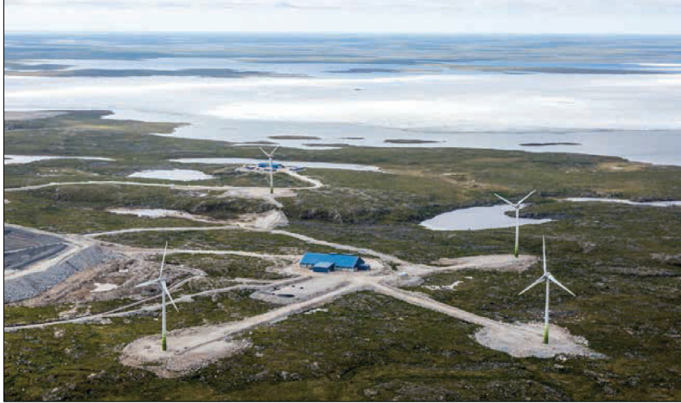
Photo 3.2-1: The Diavik 9.2 megawatt wind farm. The wind farm consists of four wind turbines.
