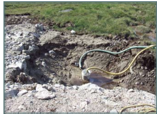
A sump installed to pump back seepage from the PKC.
