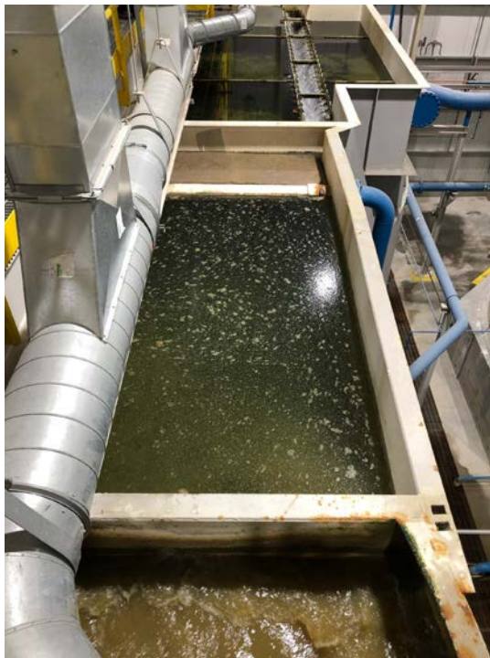
The water treatment plant is equipped to treat 90,000 m 3 of water per day, some of which is pictured in settling ponds.
