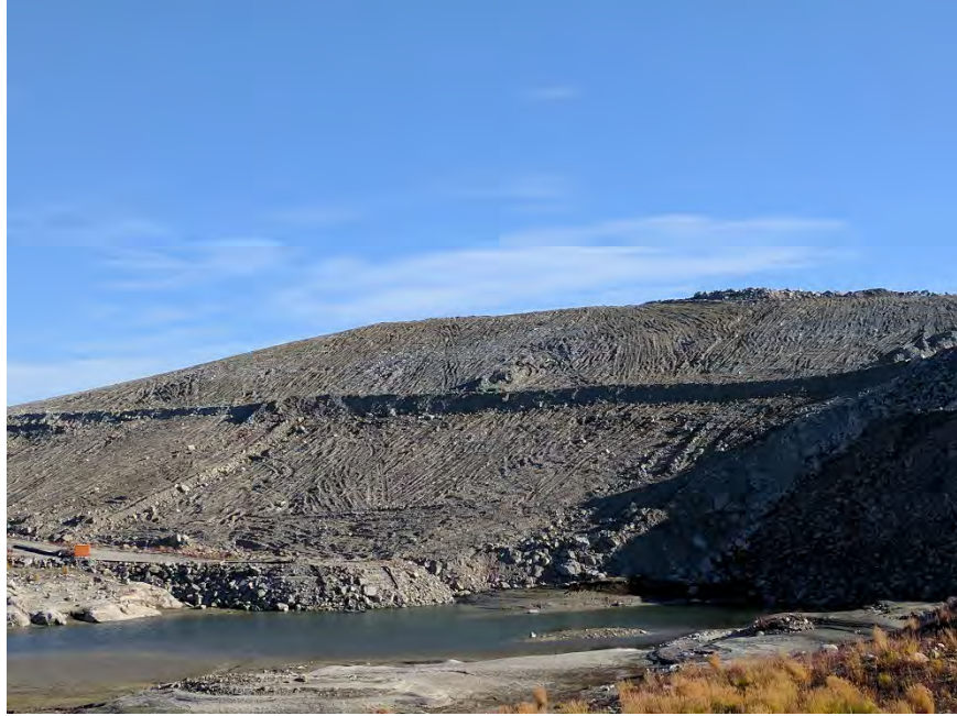
View from a distance, looking up the WRSA-NCRP that has been re-sloped.
