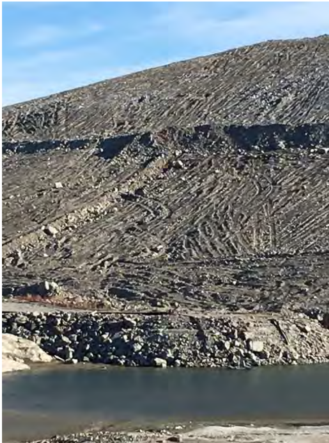
Close up view of the west side of the WRSA-NCRP, which has been re-sloped to enable cover placement and safe movement of caribou in the future.
