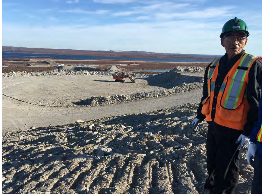
Louis Zoe stands at the top of the Waste Rock Storage Area -North Country Rock Pile (WRSA-NCRP) that has been re-sloped (at 3:1) according to suggestions made by the TK Panel, with caribou pathway in the background.
