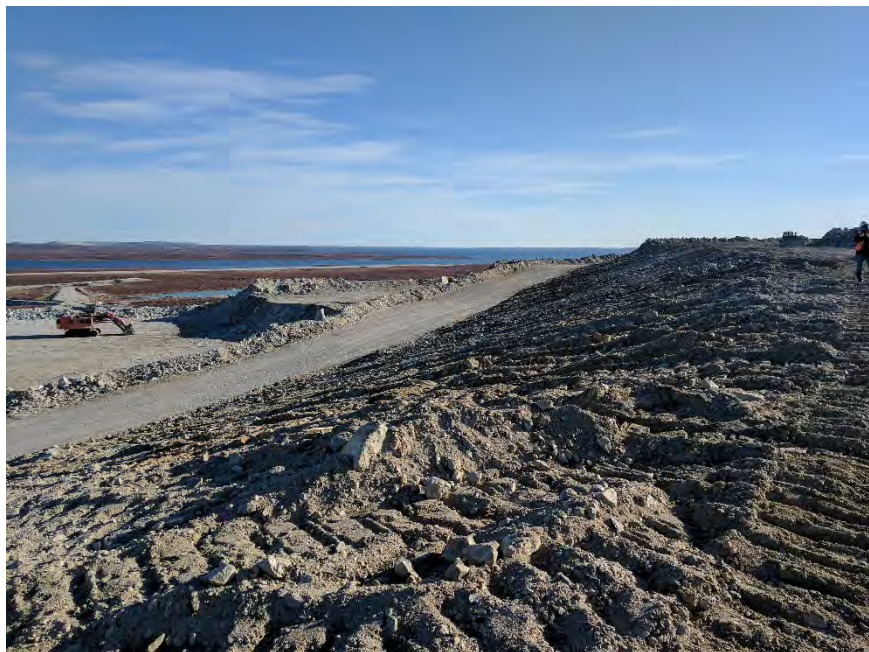
An access road for WRSA-NCRP re-sloping work has been situated in an area that will become part of the caribou walking path at closure, in accordance with design recommendations from the TK Panel.
