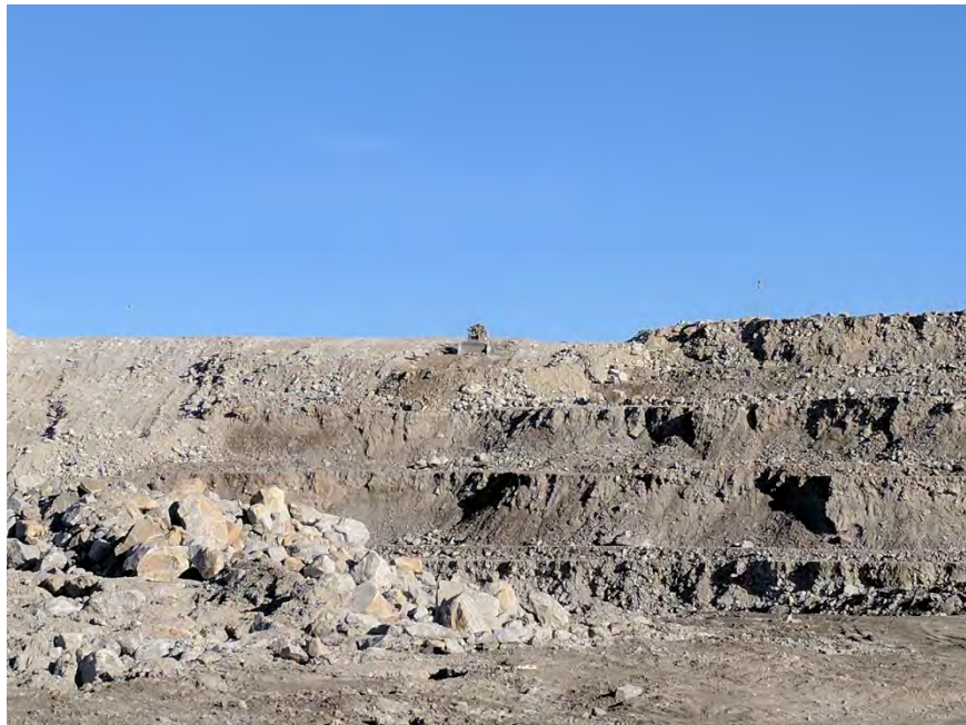
Southern flank of the NCRP, still in the process of being re-sloped.
