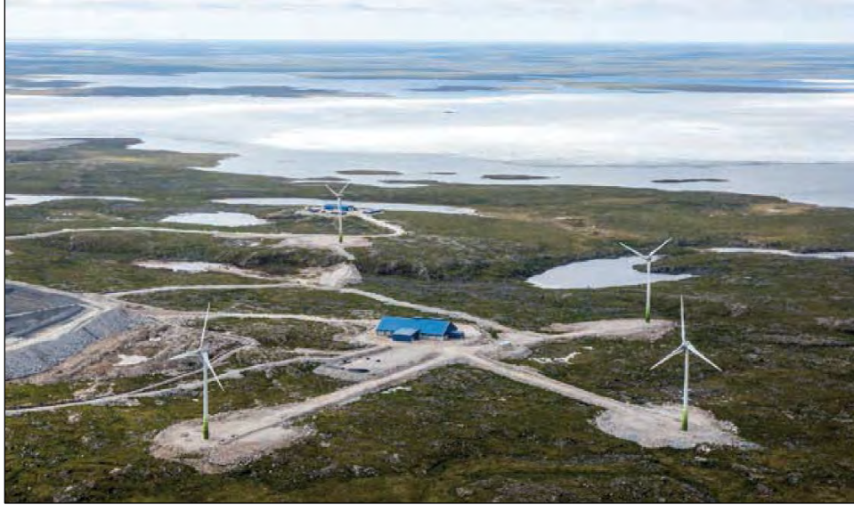
Photo 5.2-1: The Diavik 9.2 megawatt wind farm. The wind farm consists of four wind turbines.
