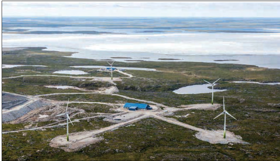
Plate 5.2-1. The Diavik 9.2 megawatt wind farm. The wind farm consists of four wind turbines.
