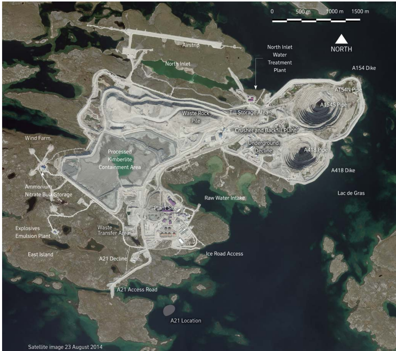
Figure 1 Diavik Diamond Mine Labelled Site Satellite Photo
