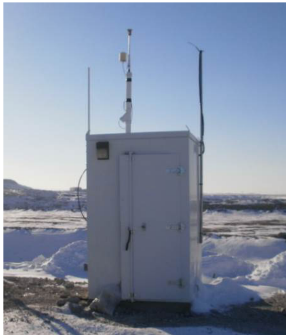
Plate 2. A154 Dike Road Location
