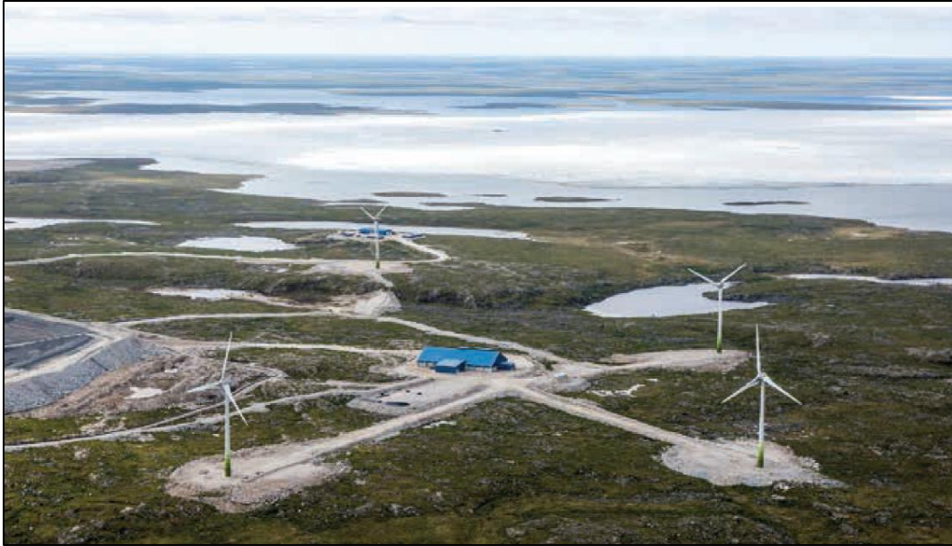
Plate 5.2-1. The Diavik 9.2 megawatt wind farm. The wind farm consists of four wind turbines. (Diavik 2015)
