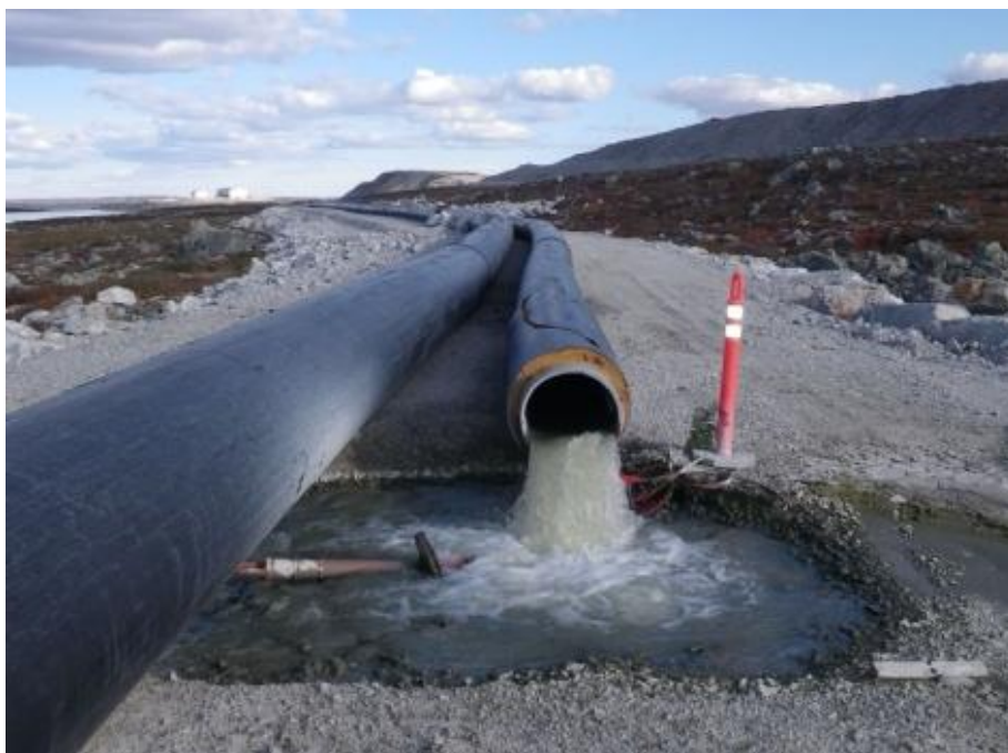
Figure 1: First discharge pipe to North Inlet from direction of NIWTP. Discharge water appears to contain light brown / grey suspended solids that settle out onto bottom sediment once discharge enters North Inlet. UTM coordinates (UTM Zone 12): 533749 easting, 7153478 northing.
