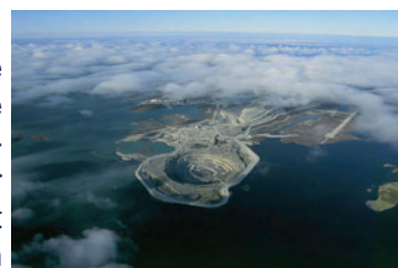
Construction of the A418 dike
