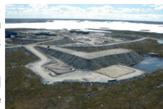
Aerial view of the pads for the test piles
