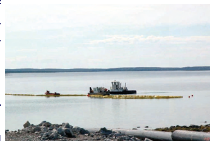
Placing the curtain around the A418 dike area
